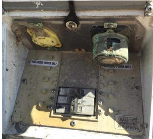
Figure 11: Typical utility pedestal receptacles
