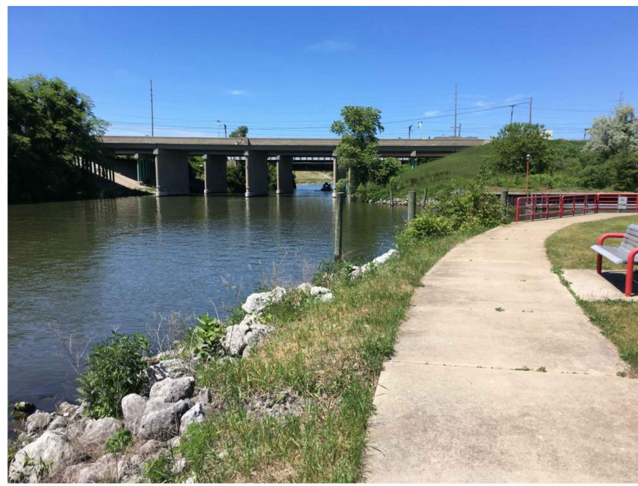
PHOTO UNDER DUNES HIGHWAY BRIDGE FOR PROPOSED NON-MOTORIZED TRAIL EXTENSION
