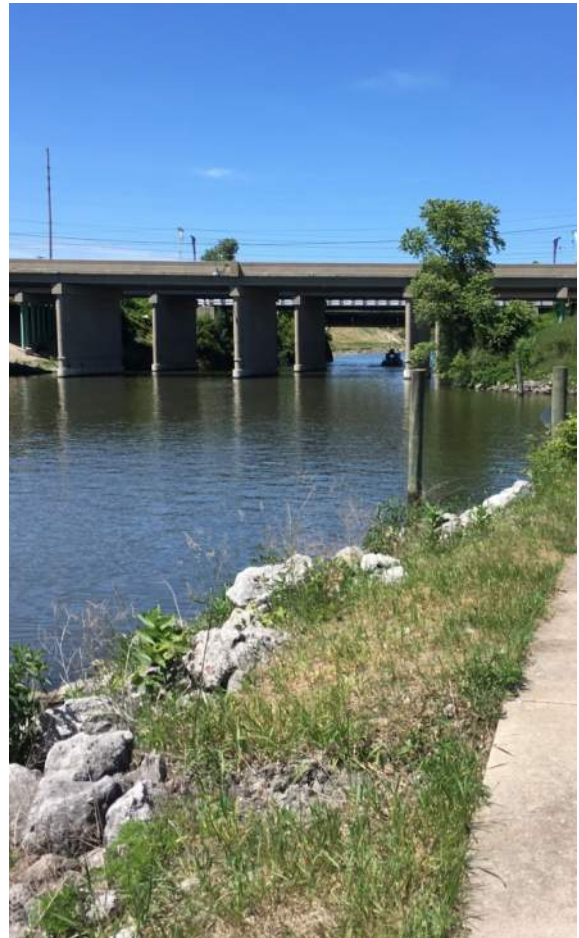
Figure 3: Dunes Highway bridge downstream of marina, looking north
