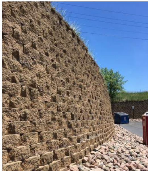
Figure 5: Block retaining wall
