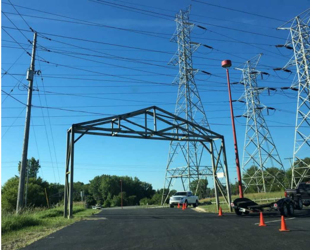
Figure 2: Overhead timber truss
