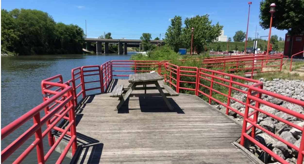
Figure 19: Fishing pier, looking north
