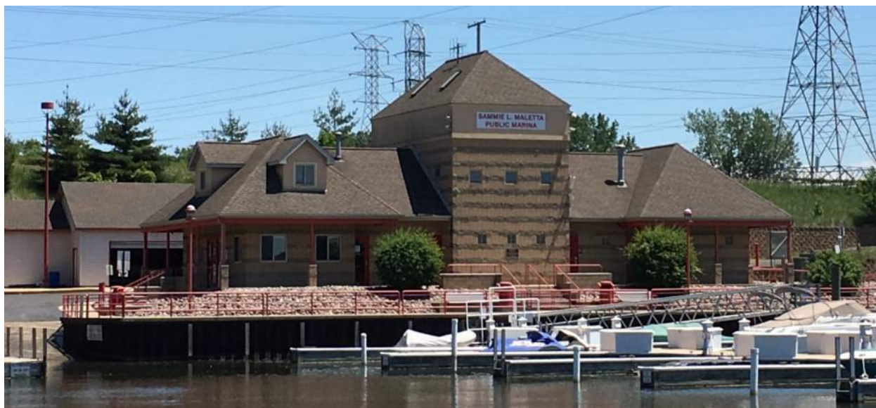
Figure 23: Marina office/support building
