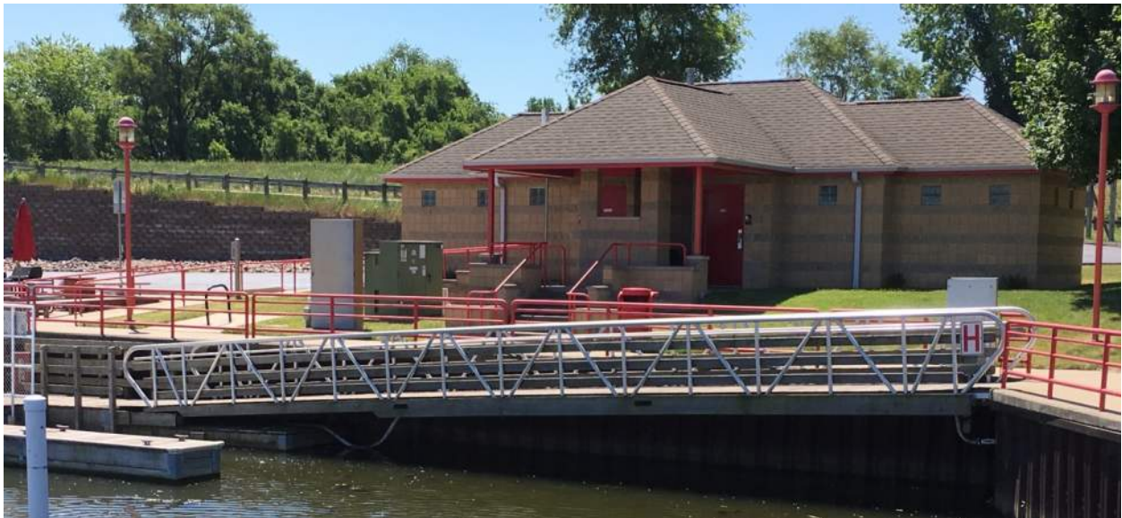
Figure 22: Restroom/shower building, looking south
