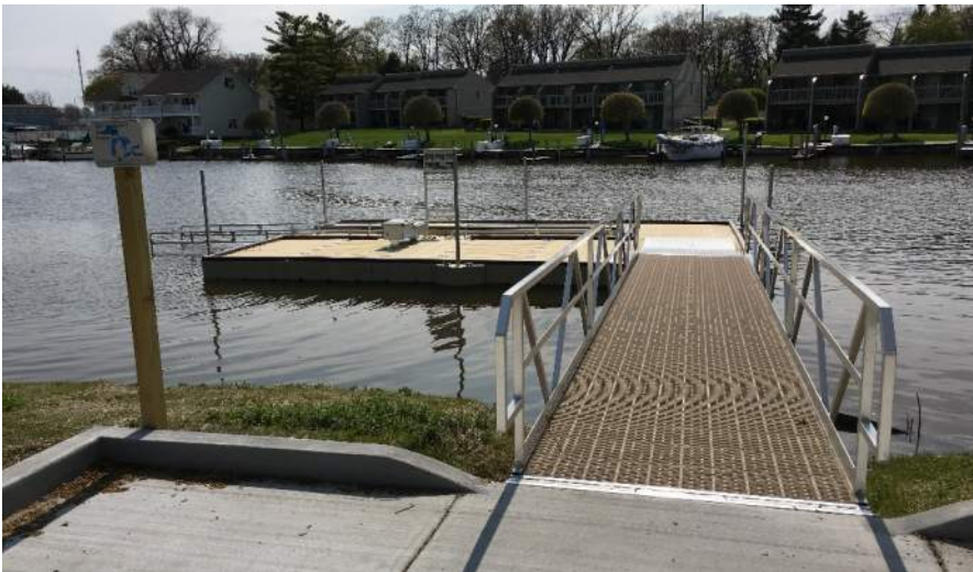
Figure 32: New accessible kayak/canoe launch, City of South Haven, MI
