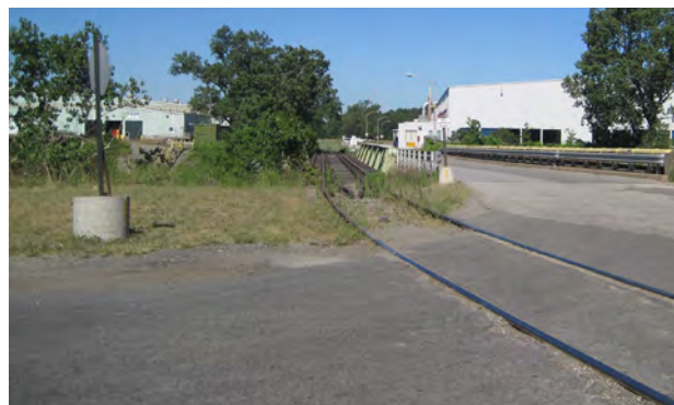
Active rail connecting U.S. Steel & Precoat Metals
