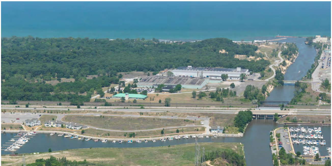
Burns Waterway (looking north to Lake Michigan)
