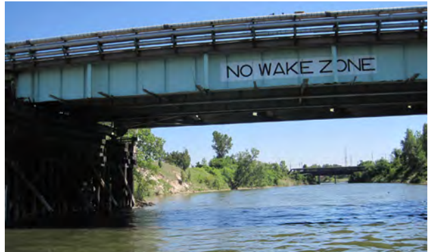
Burns Waterway at U.S. Steel bridge
