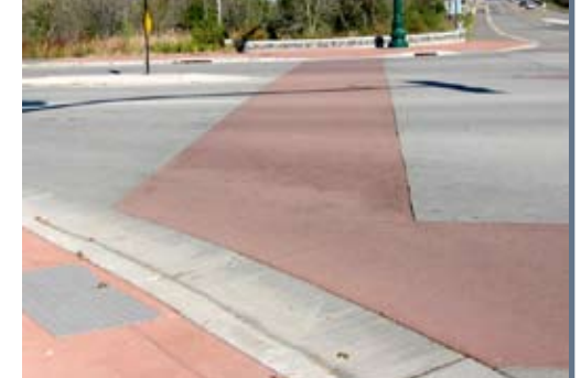
Crosswalk with highly visible colored concrete.
