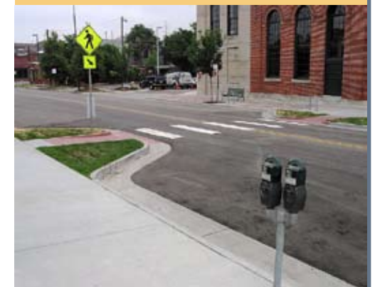
Bump outs extend the sidewalk out to the street beyond the parking spaces.
