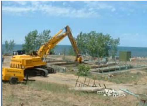
New construction in Portage.
