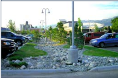
Stormwater management implemented with a parking lot rain garden.
